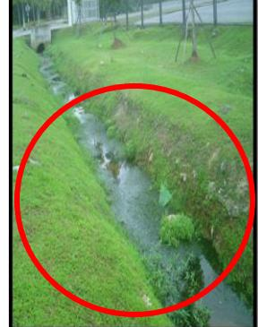
A photograph showing a drainage channel (parit) that is dirty and filled with debris, including fallen leaves and trash. A red circle highlights the debris and lack of cleanliness. |
